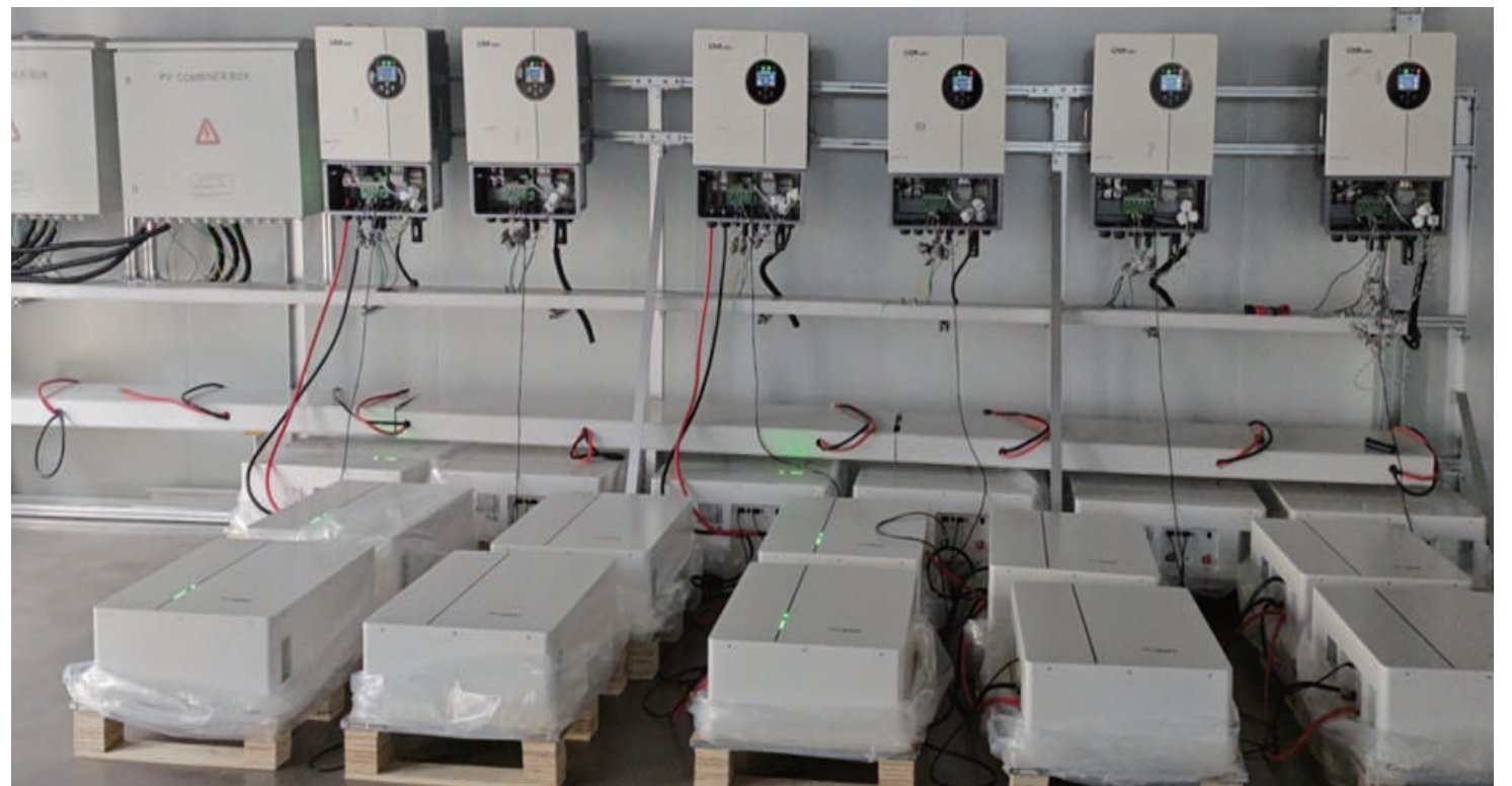
Installed capacity: 150kWh Product specification: 72kW / 150kWh Low Voltage Energy Storage System
