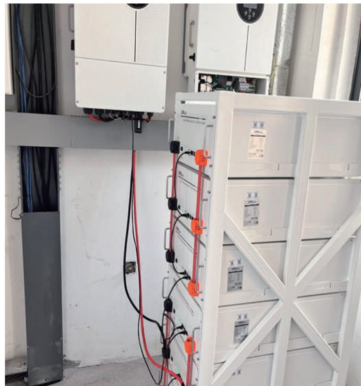
Product specification: 2 x 12kW Hybrid Inverters + 6 x 15kWh Rack Batteries
