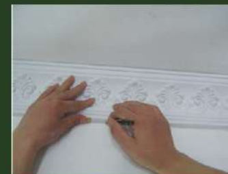
1. Establish a horizontal reference line on wall for the cornice.
