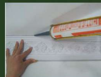
5. Apply filler to fill up gaps.
