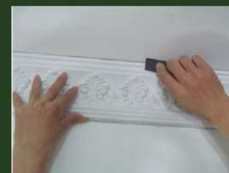
7. Use emery cloth to grind the amending place.
