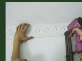
4. Using pressure gun for installing, if the wall is too strong use the steel snail.
